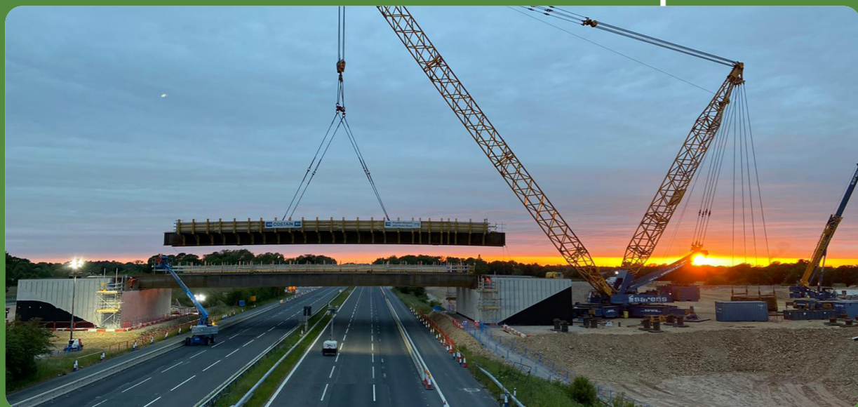
Construction of Preston Western Distributor Road
