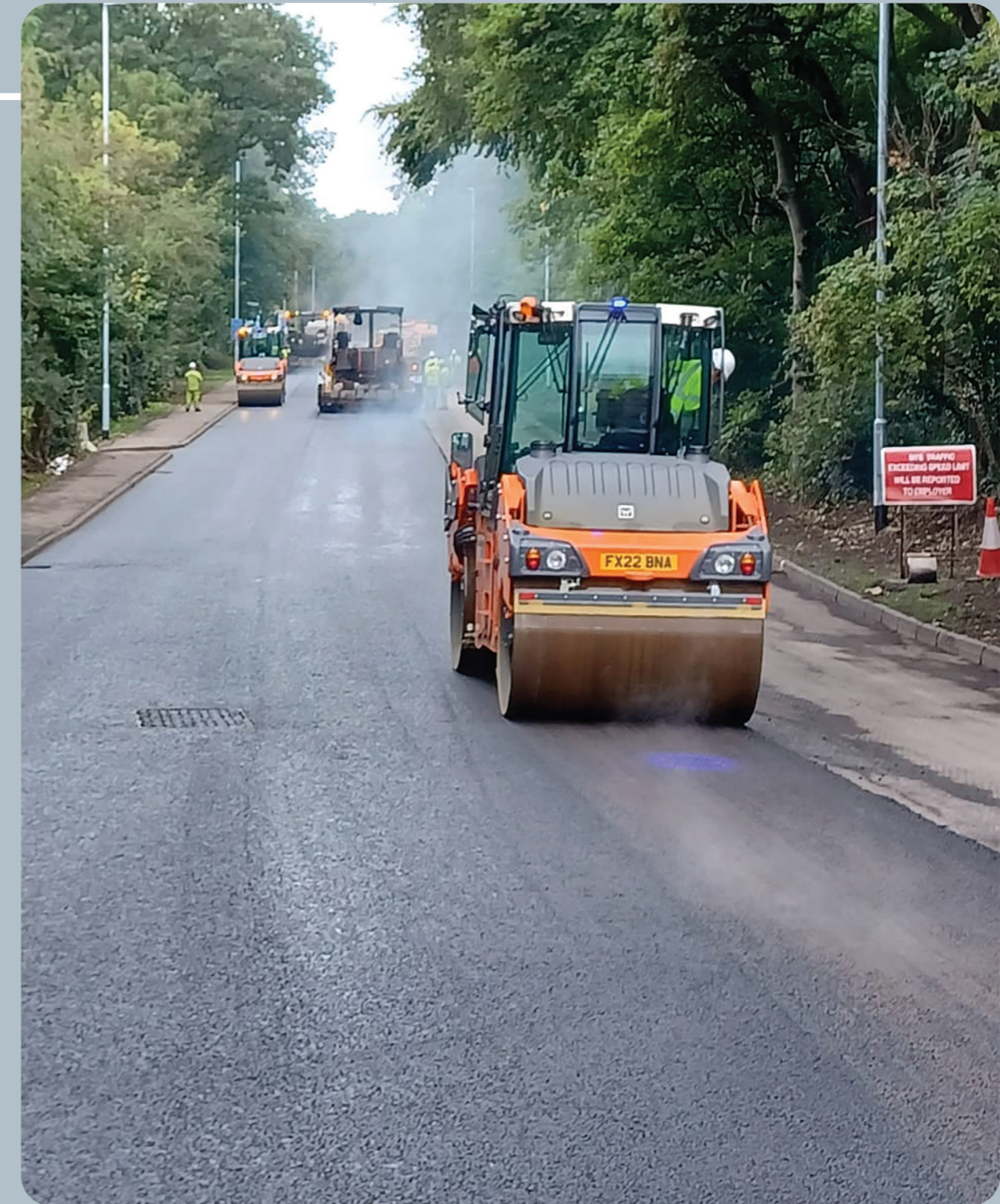
Road resurfacing on Brockholes Brow
